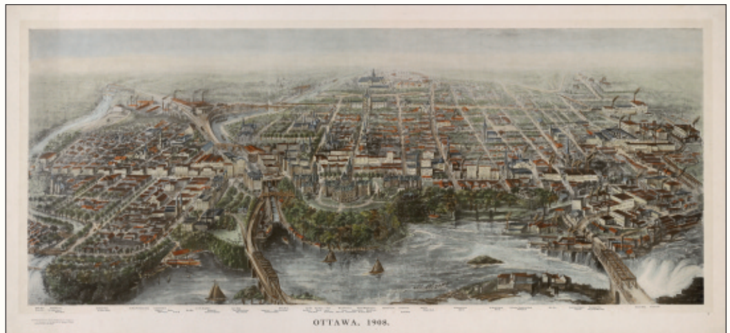
Figure 5: This view looks south over Ottawa from the Ottawa River, showing industry near the source of waterpower and major companies south of the Parliament Buildings. The Chateau Laurier and Central Passenger Station are shown several years before they were built, as was sometimes the case with bird's-eye views.
